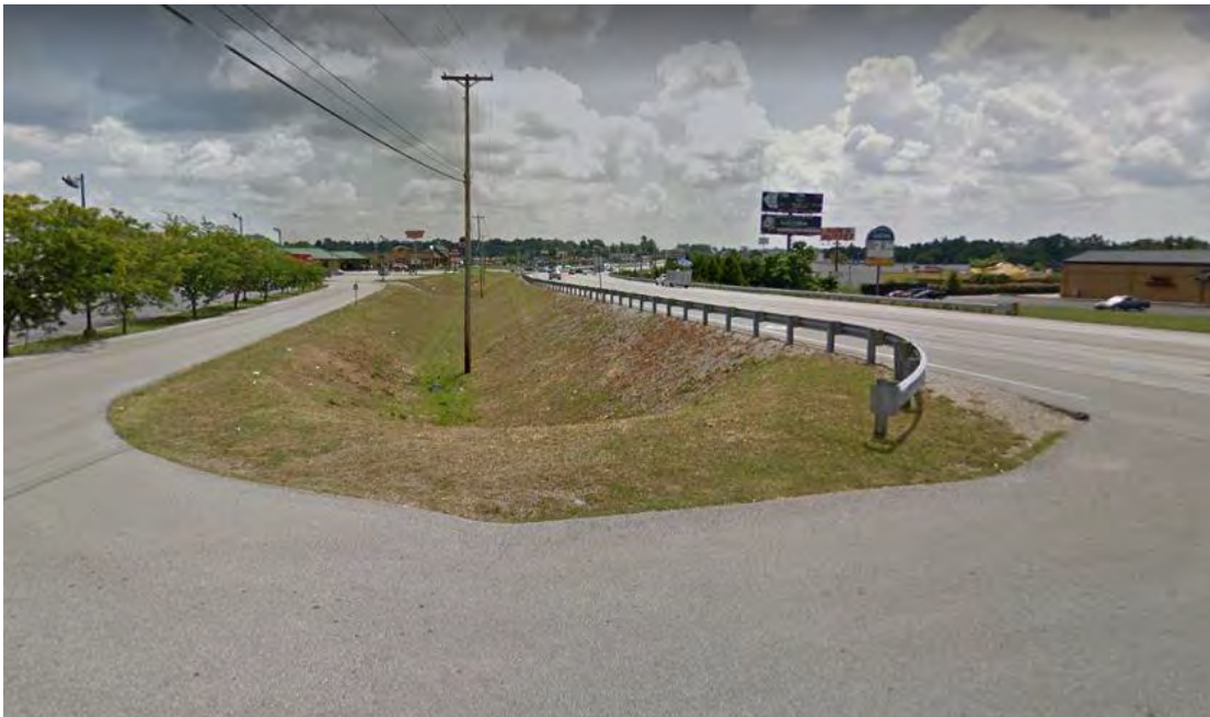
Figure 24. Point (E). Slope, grading, and drainage along north side of KY 192 facing east.
