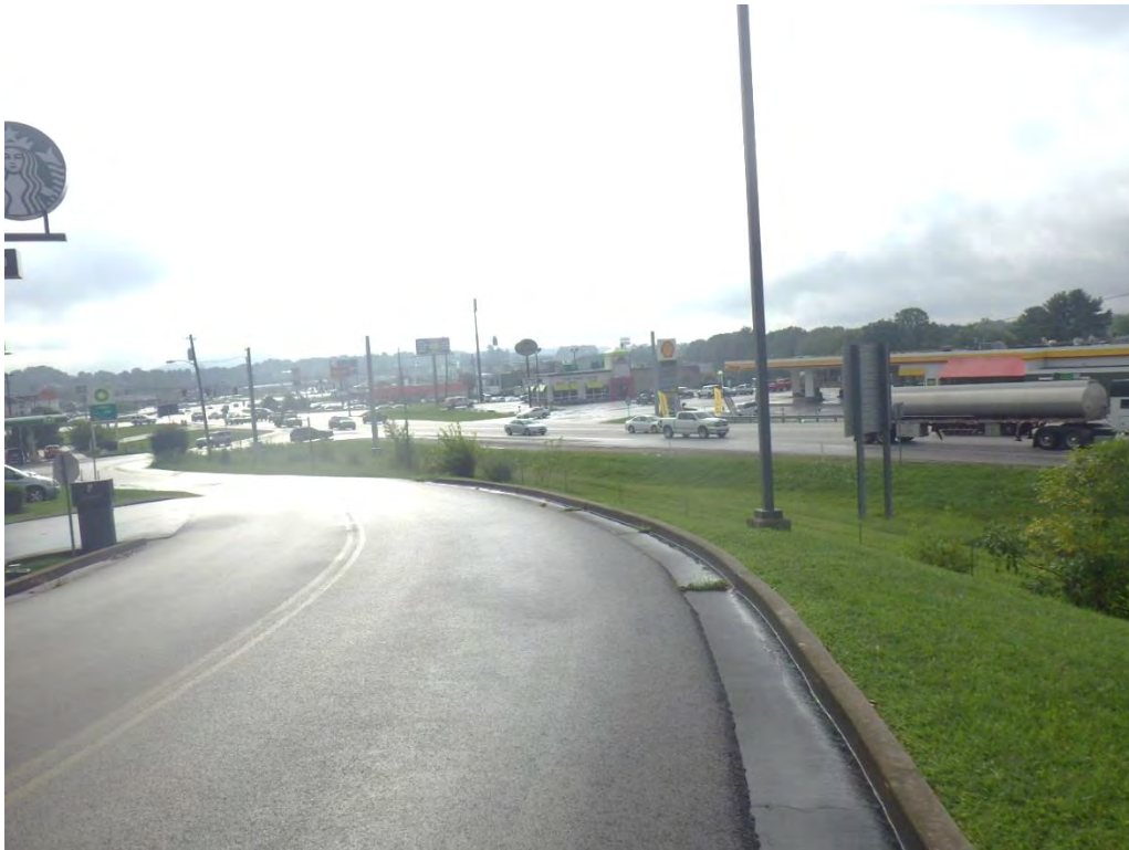
Figure 5. View to east over western edge of project APE.
