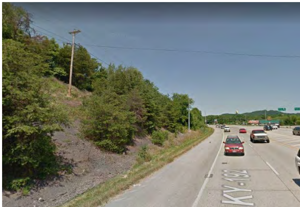
Figure 30. (Point D). Slope and drainage along north edge of KY 192.
