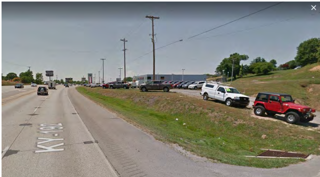
Figure 26. (Point B). KY 192 facing west showing grading and drainage along north side of KY 192.
