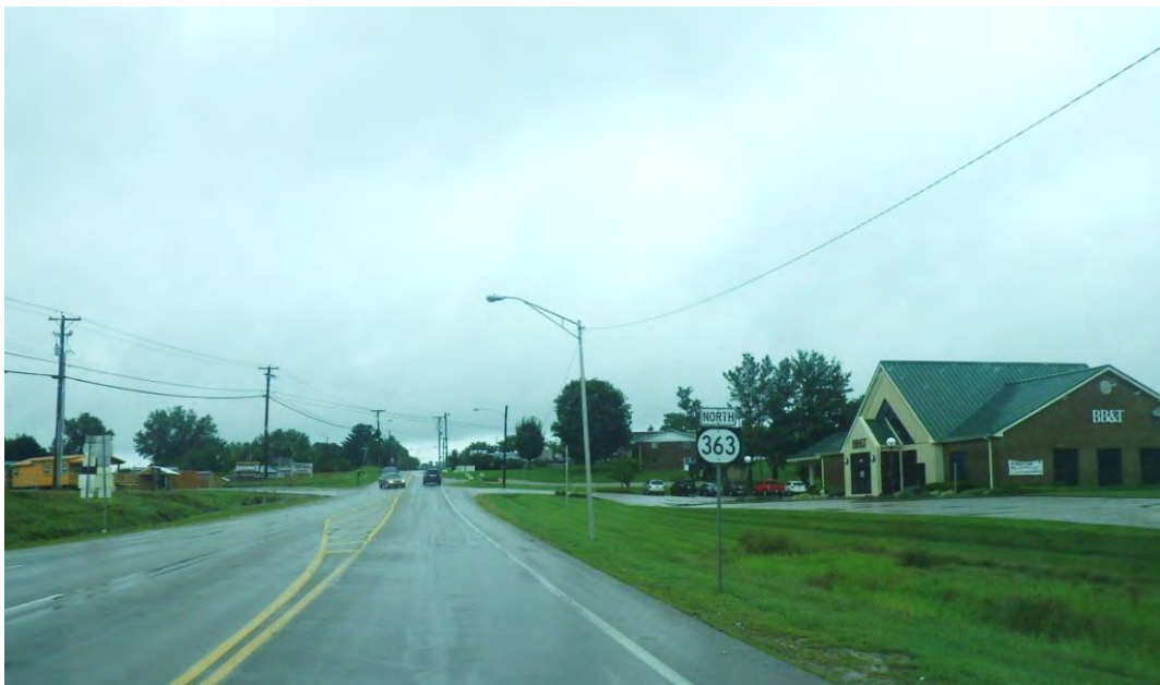
Figure 18. View to north on Hwy 363 spur of APE near the center of the project area.
