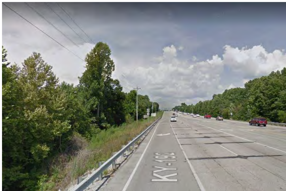
Figure 28. (Point C). Slope along north edge of KY 192 in eastern APE.
